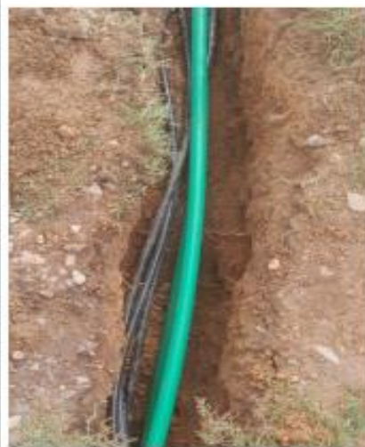
HDPE Pipe Laying
